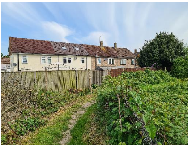
Views of rear of Nos. 73-79 Heysham Drive from public footpath
